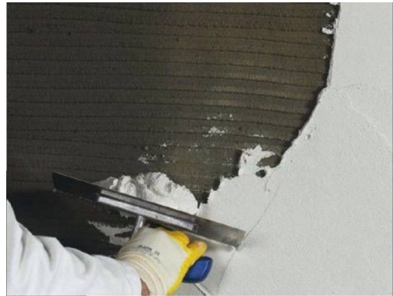
Application of plaster after MC-BondAid Plast
